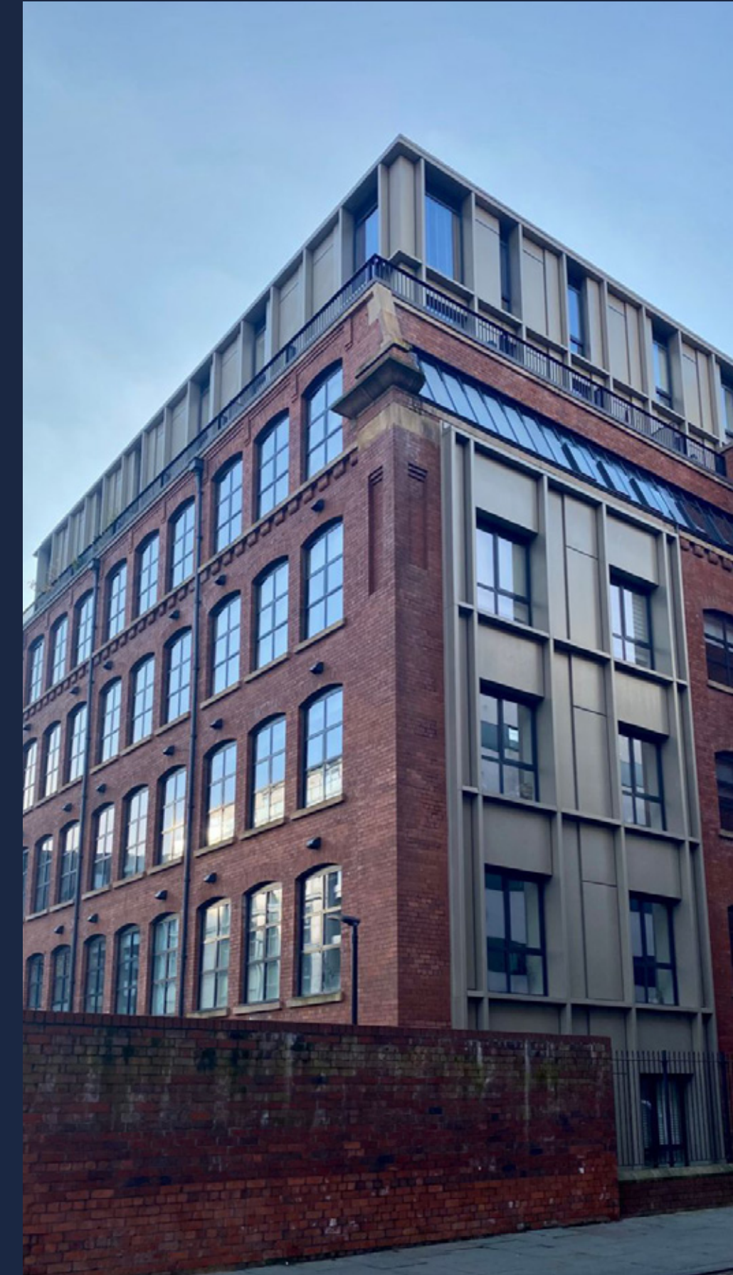
New Little Mill, Ancoats, Manchester
